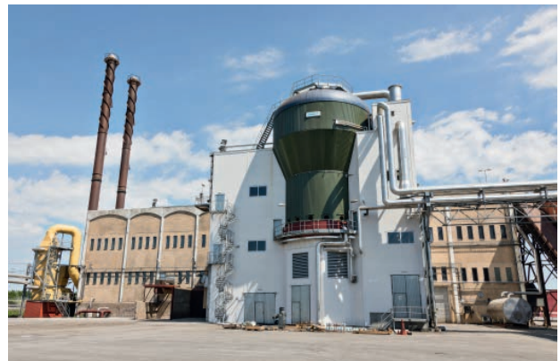
Sugar factory Örtofta: steam dryer
