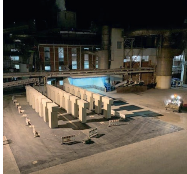
New construction of the pulp press station in Nordstemmen.
